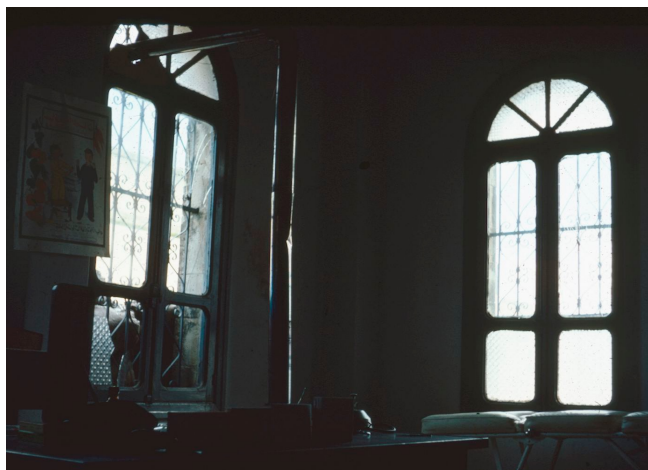
On January 1, 1978, at around 3 p.m., the clinic in Bint Jbeil was hit by nail bombs, anti-personnel explosive devices containing nails to increase effectiveness at harming victims. Windows were broken and small nails could be picked up from the floor. As this was a day off, nobody was injured. (Photo by Ebba Wergeland.)
