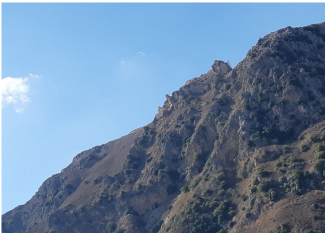
Beaufort Castle on top of the steep southern slope, November 2019. The castle was left in a state of disrepair when the Israeli forces abandoned it in 2000. In the Crusader period the castle, located on a ridge overlooking the Litani River at a height of 670 m above sea level, was an important strongpoint in the hinterland of Sidon and Tyre. With the help of the Kuwait Fund for Economic Development, a $3 million project to renovate the castle was initiated. Source: Daily Star, August 10, 2010. (Photo by Ebba Wergeland.)
