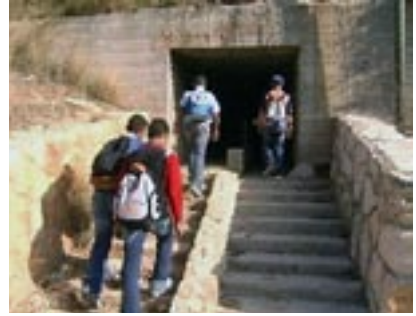
Pupils get to school via a walkway through a drainage hole.
